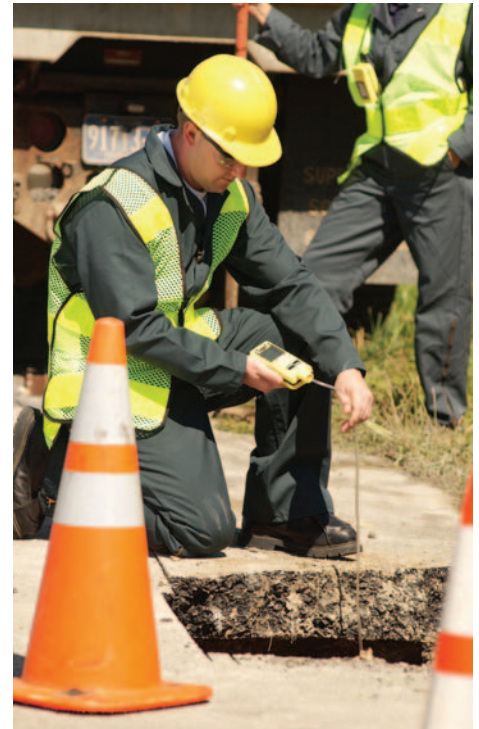
Photo courtesy of Industrial Scientific Corp., Oakdale, Pa.
